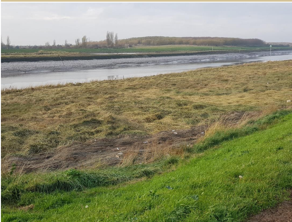
Plates A.1.4 to A.1.8 Debris within saltmarshes along The Haven (taken in November 2021)
